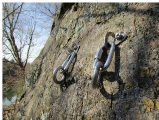
Figure 4. Expansion bolts with quick links and steel rappel rings.
