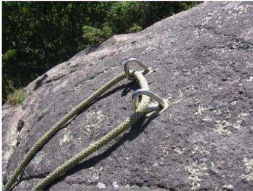
Figure 1. Glue-in bolts.
