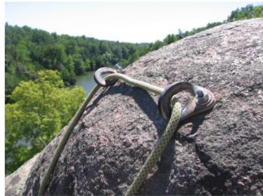
Figure 2. Expansion bolts with ratchet hangers.
